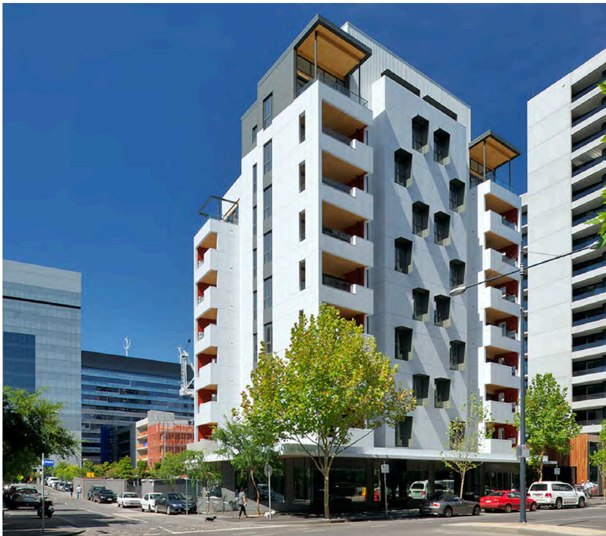
Fortè residential apartment building in Melbourne constructed using engineered wood products (EWPs).
